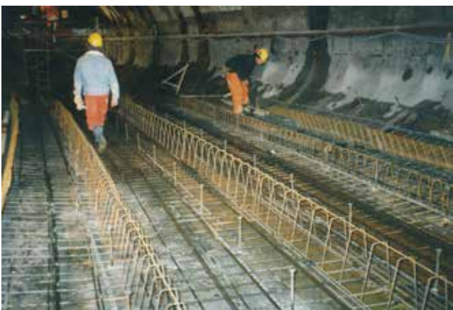
BKW Tunnel BKW tunnel
